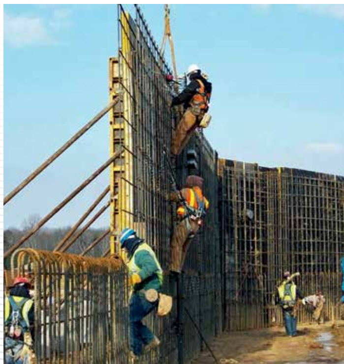
Wall being constructed around the RKB.
