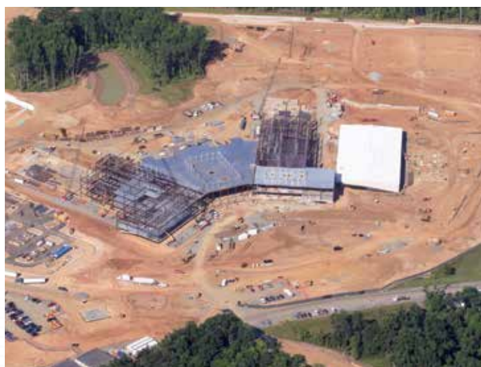
Aerial view of the RKB construction site.
