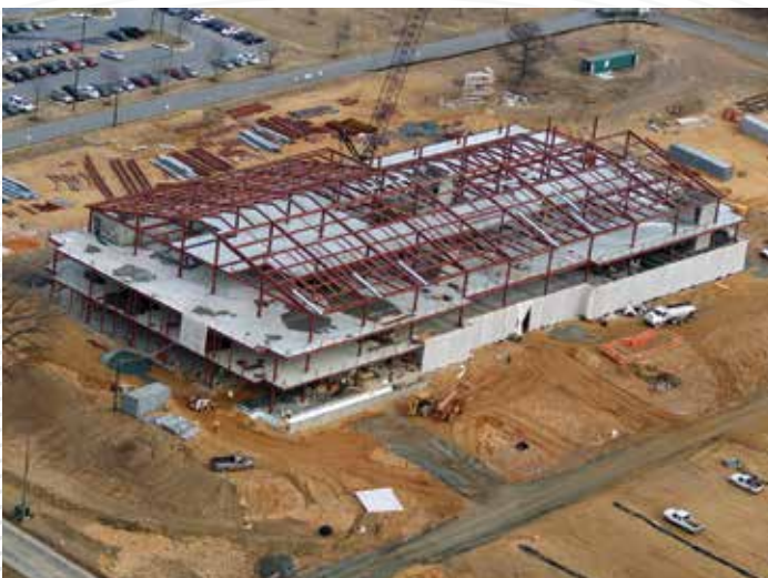
Aerial view of the construction site for the Fort George G. Meade building in Maryland.
